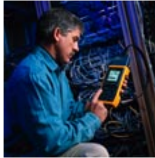
Certification testing of structured cabling system
